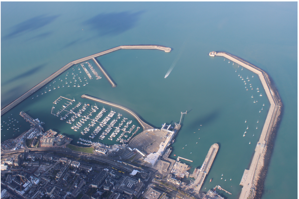
Figure 5.1.3: Aerial Photograph of the harbour, 2014 (Source: Sgt. Paul Maguire, Irish Air Corps)
