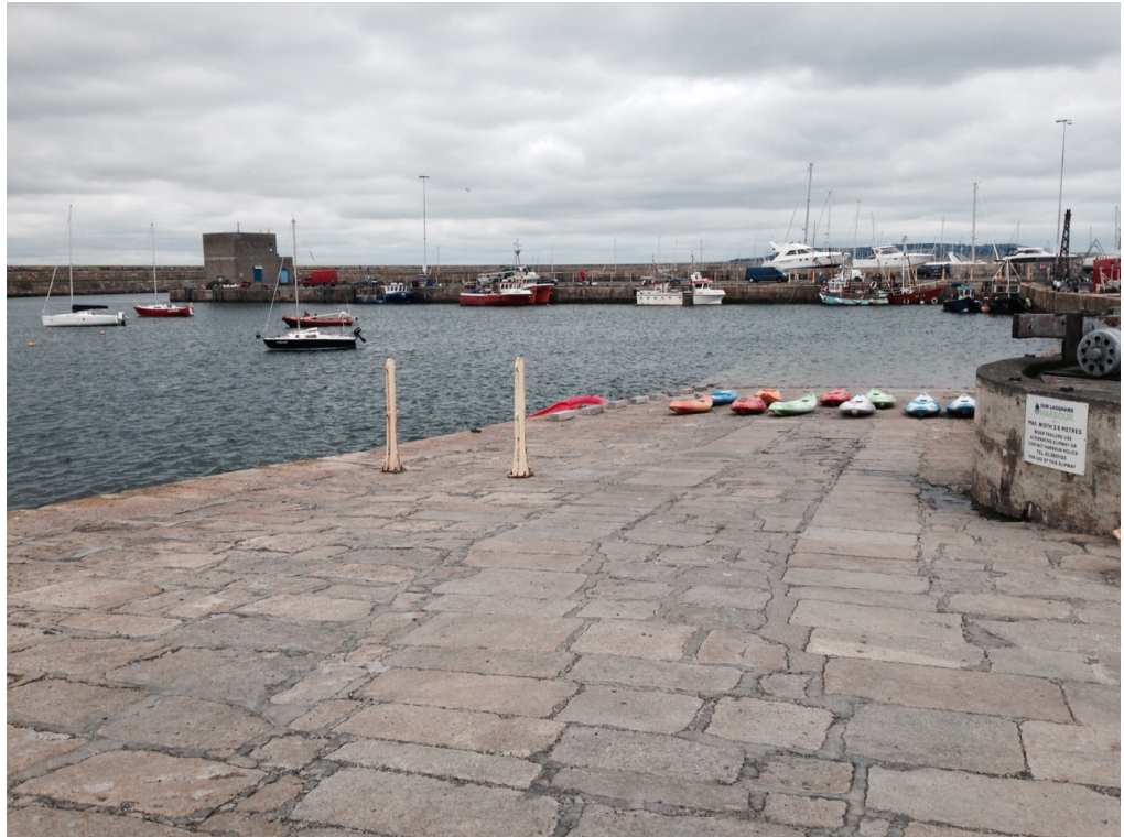
Figure 5.1.16 – Public Slipway in the Coal Harbour
